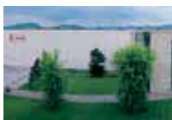
The New Factory
